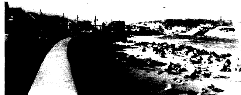
Figure 3.4 Photo of seawall
