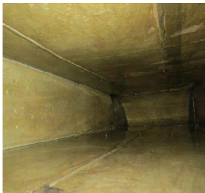
Before and after ductwork photos
