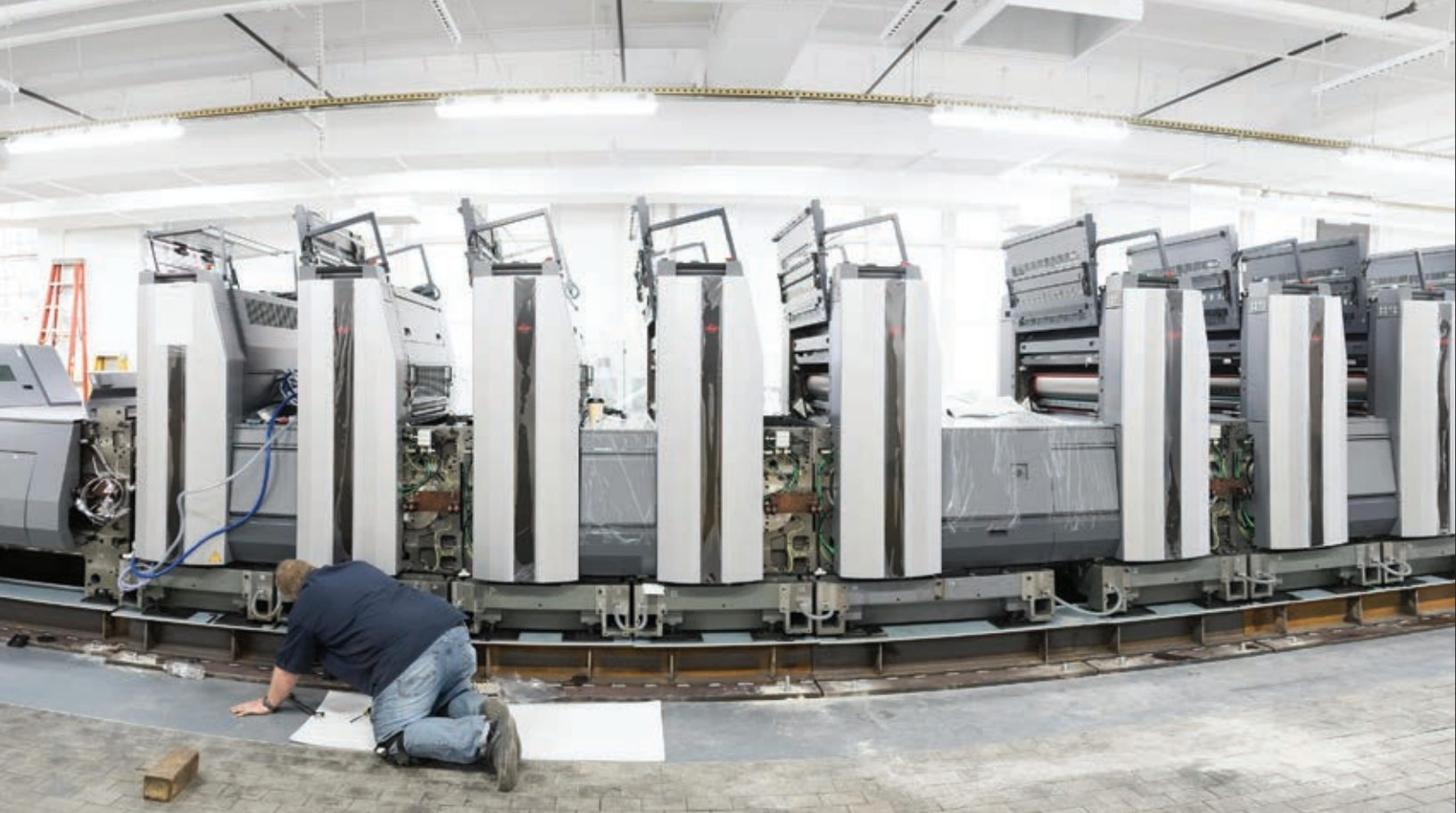
The new 8-color press being installed.
