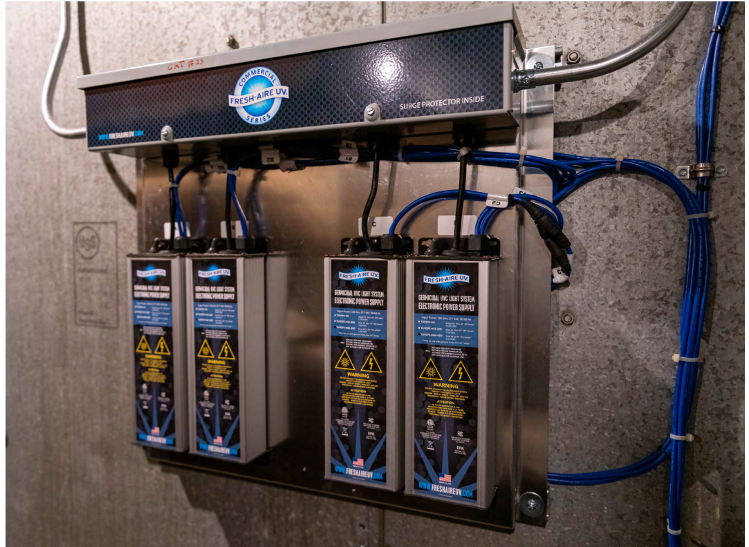
GPO's new UV lighting system is a preventative measure to protecting the air in the building.
