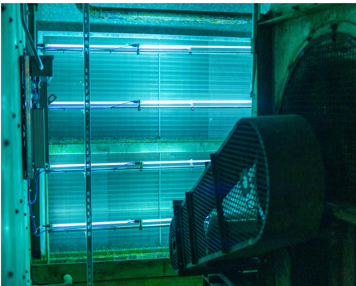
UV lighting is used as a means to kill germs like bacteria and viruses.
