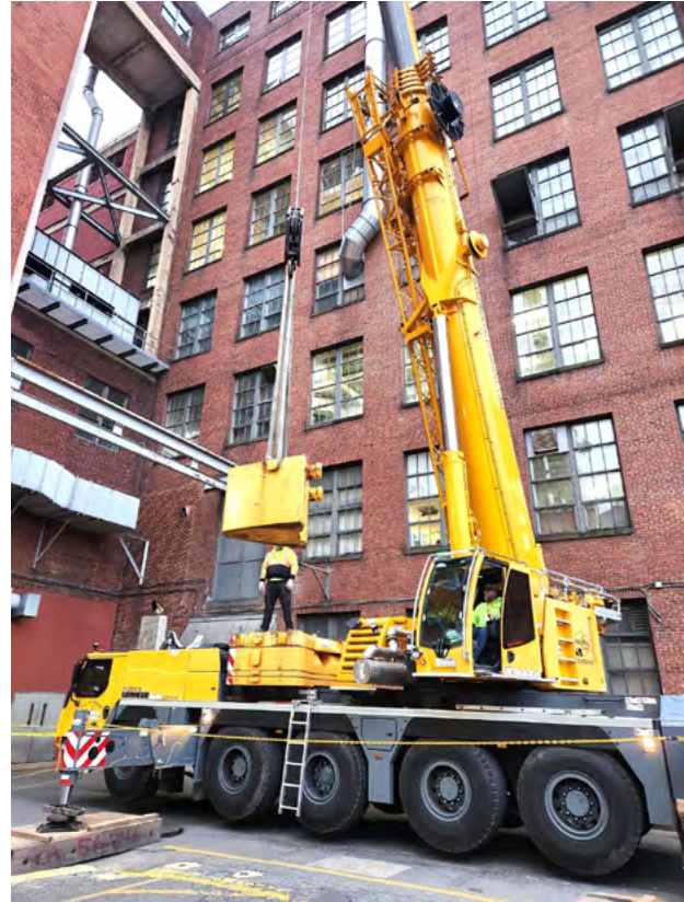
GPO removes Group 86 presses as part of continued modernization of its Plant Operations.
