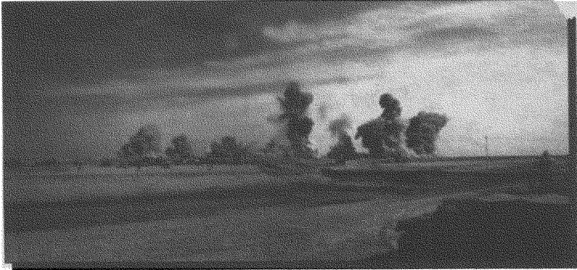
Figure 5. Demolition of bunkers at Khamisiyah, 4 March 1991.
