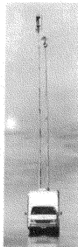
HELP ON WHEELS Trucks with cell transmitters were rolled out to restore service to Houston and other areas affected by Hurricane Ike.
