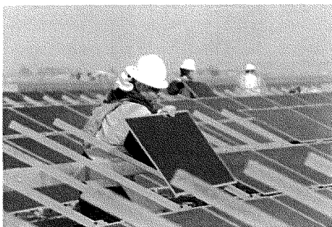
Workers install First Solar panels in Blythe, Calif. (Photo: Business Wire)
