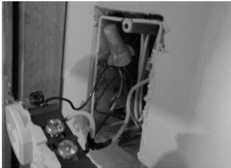
Photo 8—View of another outlet where the ground wire has corroded and turned black
