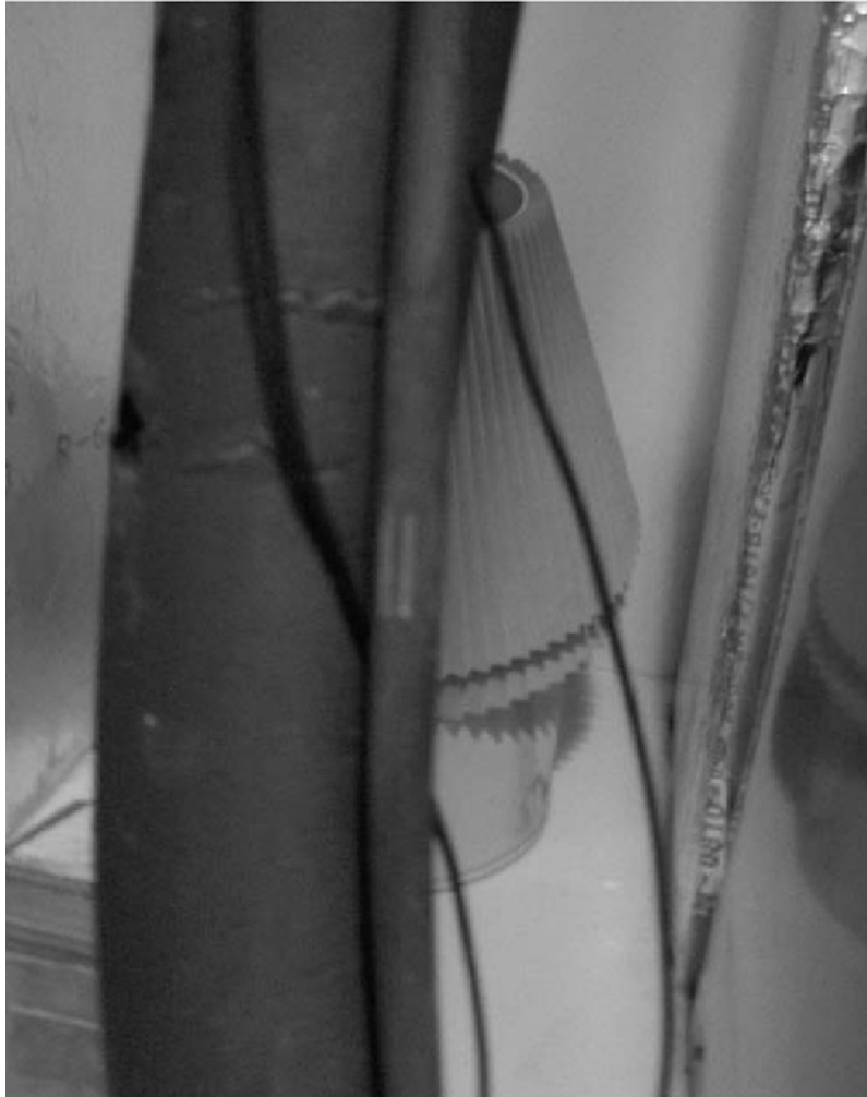
Photo 4—Close up view of the copper wire that runs alongside the air conditioning unit where it has turned black
