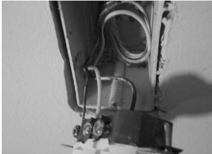
Photo 8—View of another outlet where the ground wire has corroded and turned black
