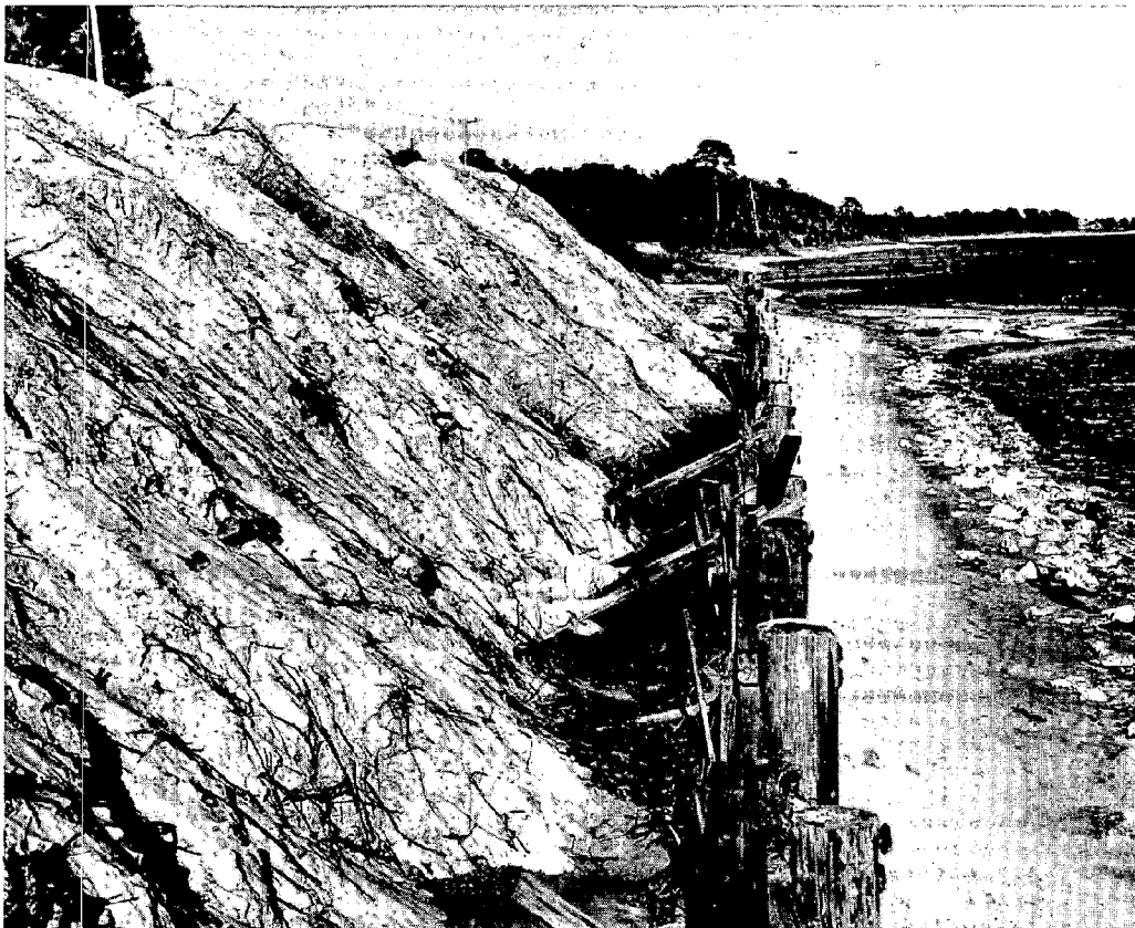
Figure 5. Attempts to extend the land into water bodies with fill and bulkheads should be avoided; there will be continuous maintenance needs and often washouts, with damage to roadways and structures. (Photo from Apalachicola Bay, Florida, by John Clark.)
