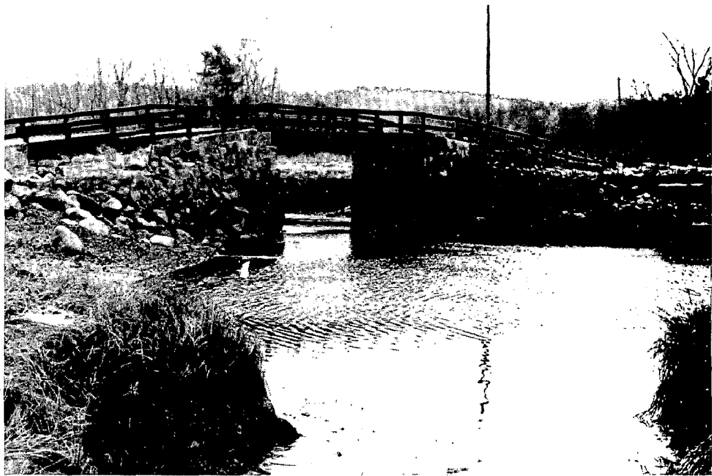
Figure 16. Bridge abutments that encroach on watercourses reduce water flow and degrade the coastal ecosystem. (Photo by John Clark.)
