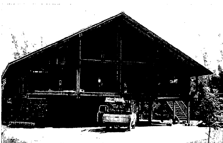
Figure 11. A house elevated on piles for protection against coastal flooding (Sanibel, Florida). (Photo by John Clark.)
