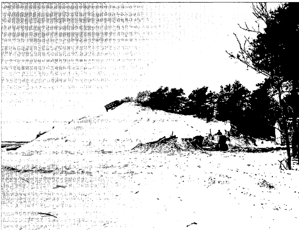
Figure 4. Excavation of sand dunes to obtain fill, level the land surface, or provide a view should be prohibited in most cases to protect the shoreline, structures, and human life during storms and floods. (Photo by John Clark.)
