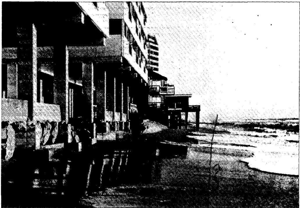
Figure 12. At Ocean City, Maryland, condominiums are still built on the beach, even though existing structures are being undermined by winter waves. (Photo by Steven Leatherman.)
