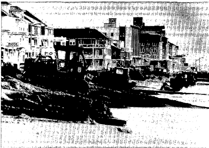
Figure 13. Ocean City, Maryland, uses bulldozers to push beach sand against failing foundations and bulkheads each winter in a futile attempt to correct the mistake of building too close to the ocean; a hurricane striking here will cause extraordinary damage. (United Press International Photo.)
