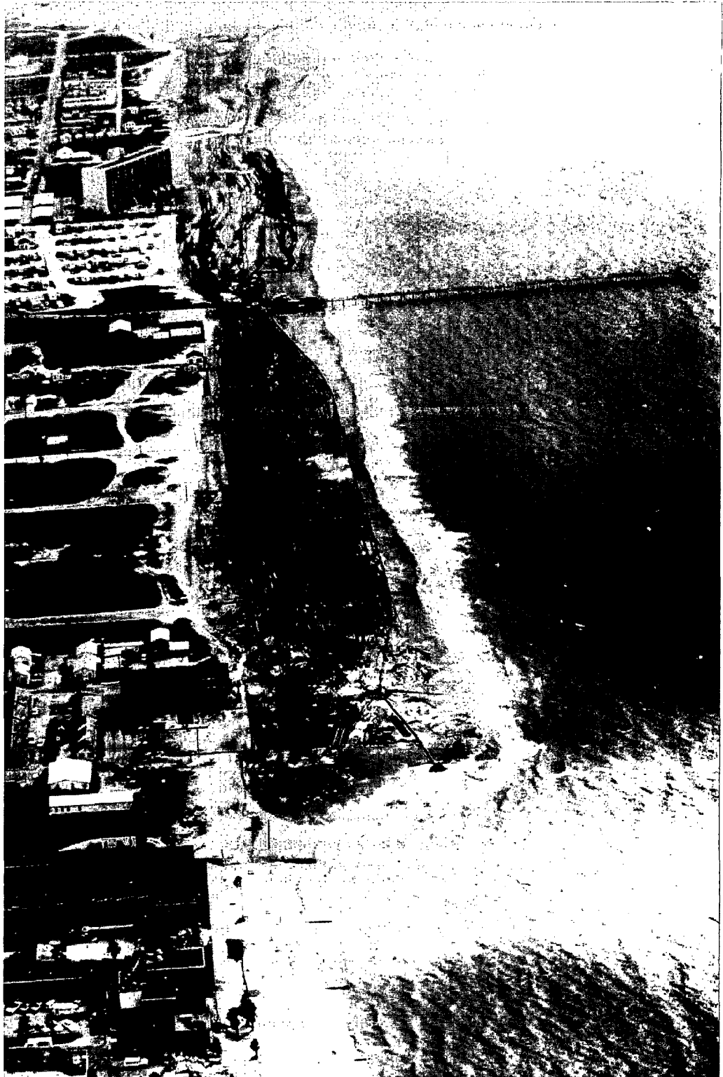
Figure 15. The North Beach at Corpus Christi, Texas, in the summer of 1977, during the dredging and spreading operation of a beach restoration project by the Galveston District, Corps of Engineers. Sand for the base was dredged from Corpus Christi Bay, with cover sand trucked in. (Photo from U.S. Army Corps of Engineers, Galveston District.)
