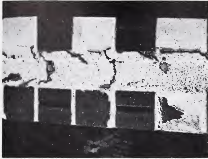
Figure 3 Section of improperly consolidated high lift reinforced grouted brick masonry wall. Wall has been rotated on its side and saw cut for visual purposes. Note the separations within the grout space.
