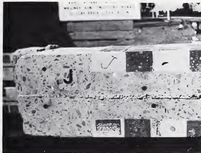
Figure 4 Section of properly placed high lift reinforced grouted brick masonry wall and foundation.
