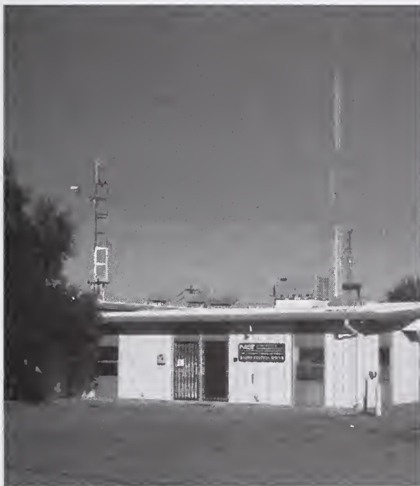
Figure 1.14. View of WWVB building.
