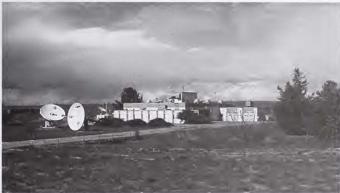
Figure 1.6. The WWV transmitter building.
