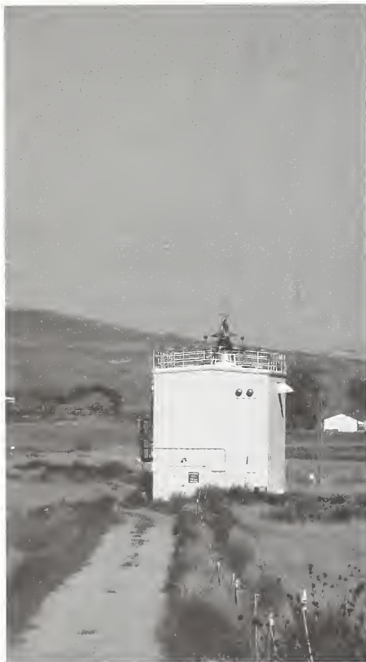
Figure 1.15. WWVB helix house.
