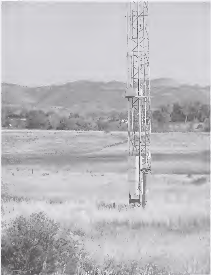
Figure 1.21. Tower counterweight.
