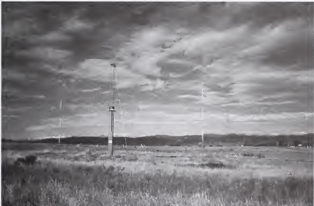
Figure 1.10. The 15 MHz antenna at WWV.
