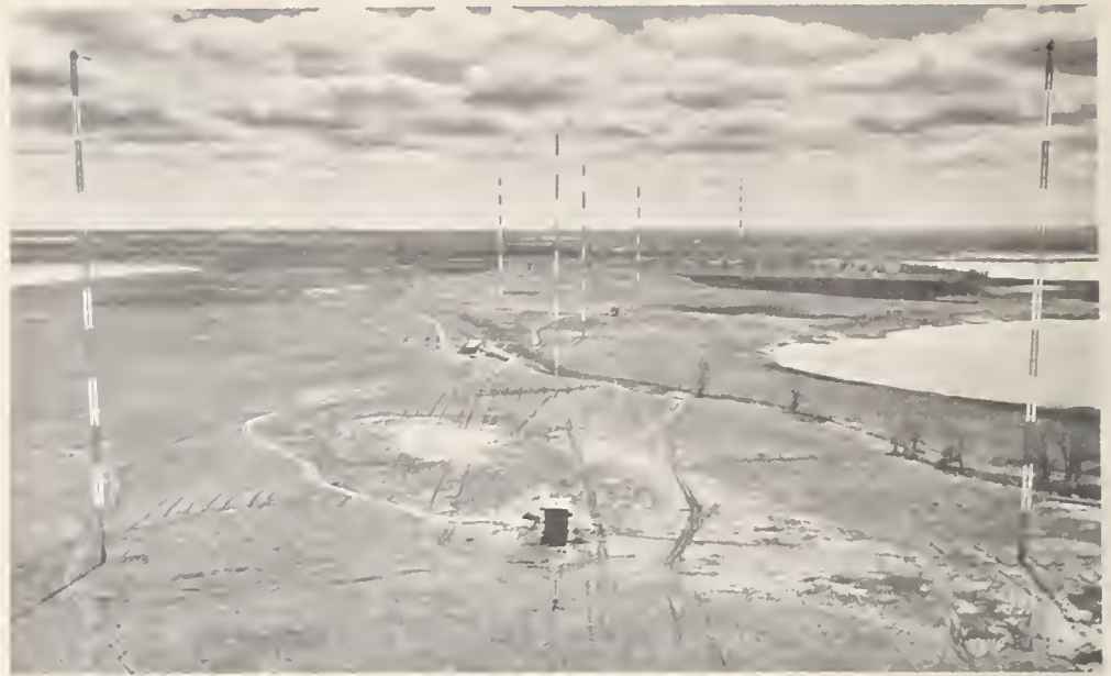
View from halfway up one of the 400-foot towers supporting antennas for the new LF and VLF standard frequency transmitting stations at Fort Collins, Colo. The "helix house" ( center foreground ) contains the helical tuning device for the antenna. Furrows show the grid pattern of the ground wires. (See p. 53.)
