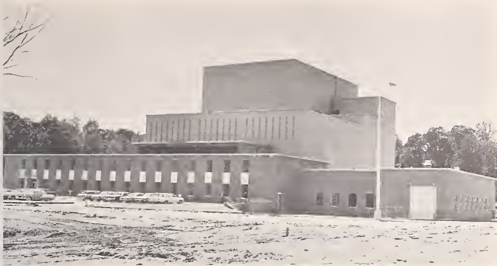
The Engineering Mechanics Laboratory at the new NBS site in Gaithersburg (Md.) is now being occupied by the first working groups to move to their new quarters. (See p. 21.)
