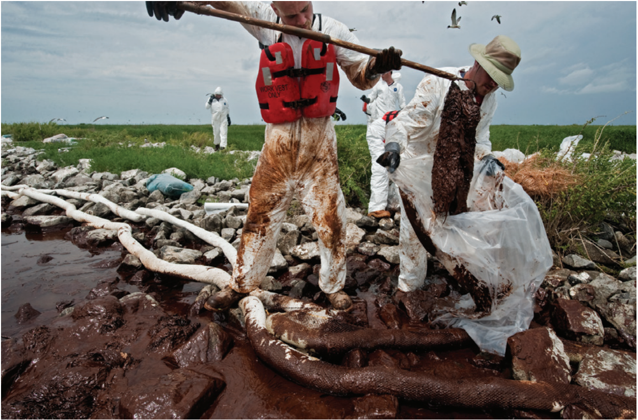
Dirty job, a cleanup crew bags oil-absorbent polypropylene “pom-poms” near a bird rookery in Louisiana. Containment booms snake past their feet. By August, cleanup efforts had generated some 40,000 tons of solid waste. Overall response to the huge spill posed unprecedented challenges to both government and industry.
